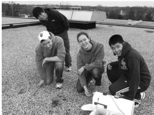
Figure 5. GBS students install GPS receiver on the school's roof.
